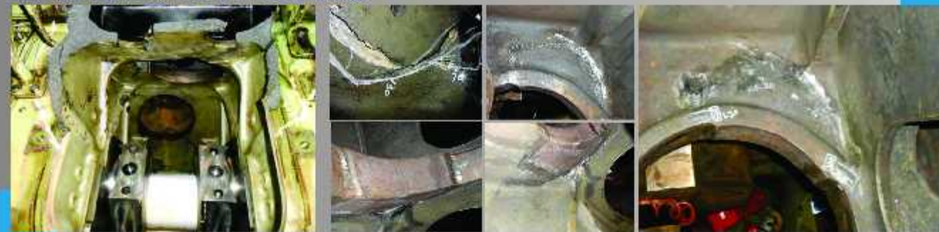
TIRE KILN CRACK REPAIR (PT SEMEN INDONESIA, TUBANI)
