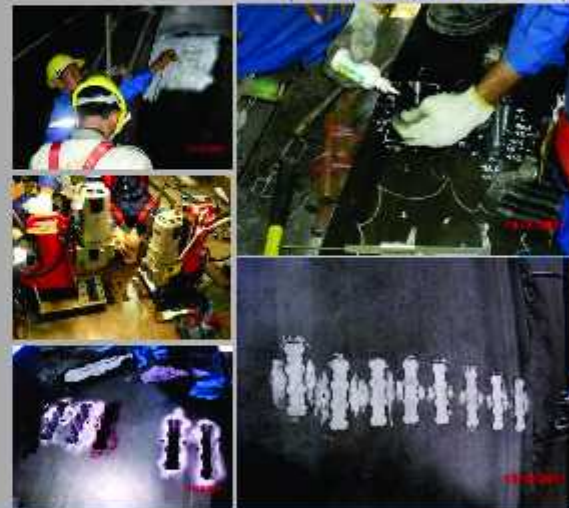
TIRE KILN CRACK REPAIR (PT SEMEN INDONESIA, TUBANI)
